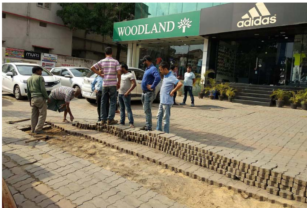
Construction of public bicycle sharing system in Ranchi
