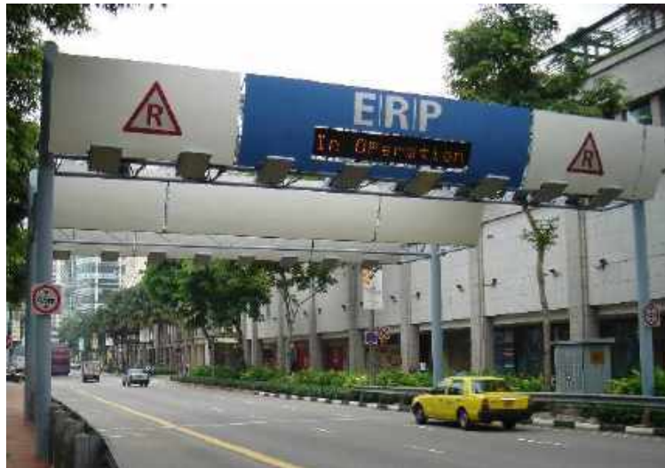
Figure 38 Gantries equipped with both DSRC and ANPR cameras in Singapore to charge vehicles and detect violations respectively
